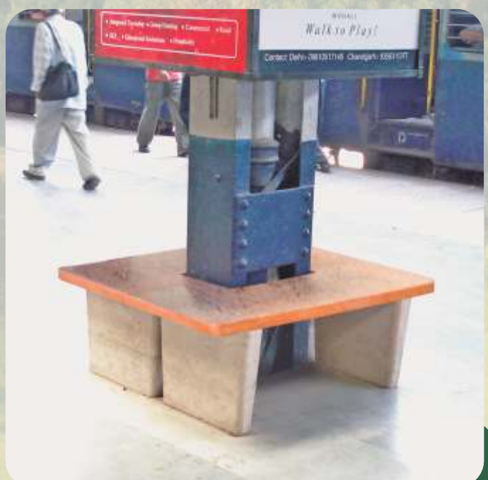
Concrete Bench for placing around the pillars. Terrazzo Finish
